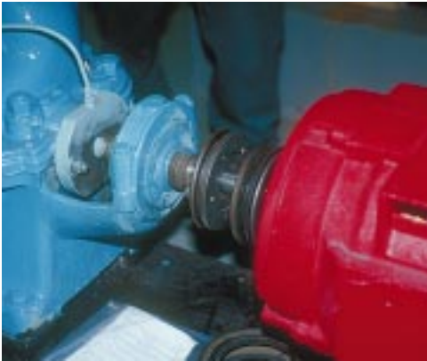
New motor installation.
