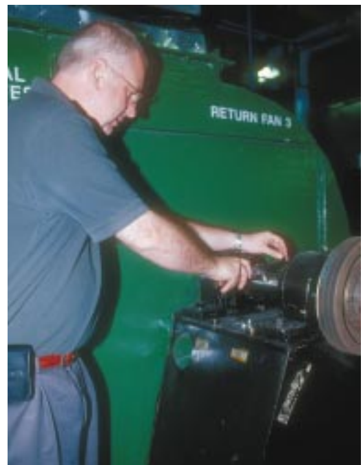
Measuring for bearing replacement.
