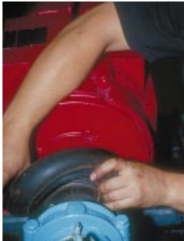
New coupling Installation.
