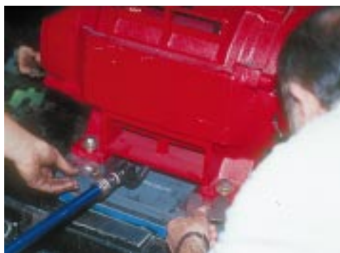
Motor alignment and shim installation, as dictated by the latest technology.
