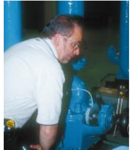
Installation of alignment equipment.
