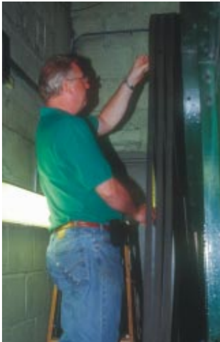
Measuring a companion pulley and variable pitch sheave combo for replacement.
